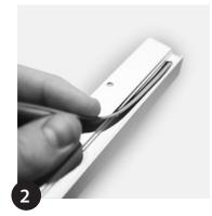
Conceal wiring in channel (threading through hole in mounting surface if required).
