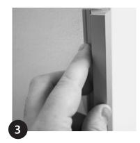
Conceal wiring in channel passing through hole in mounting surface – if required. Press firmly in position.
